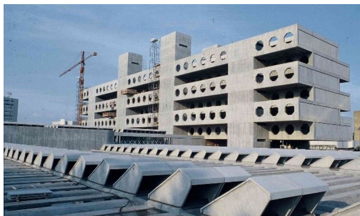
Obra Hospital SARAH Brasília
